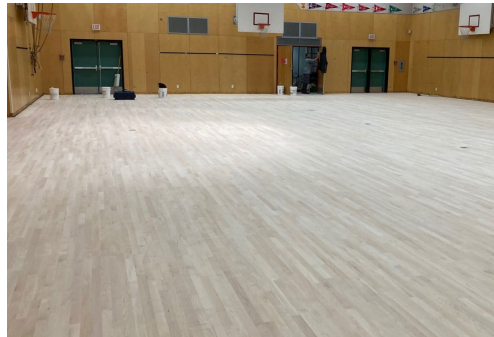
Week two Sanded and ready for varnish
